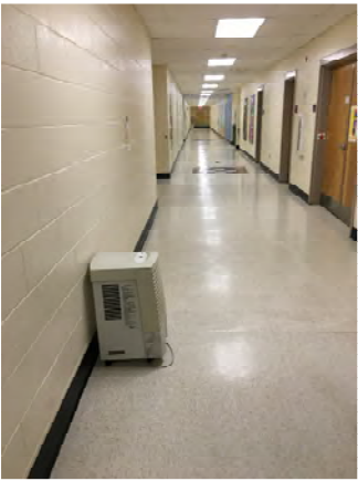
Basement flooring, water vapor & concrete topping replacement at Northern Elementary
