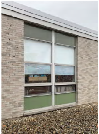
Window Replacement & Abatement, includes security film at Central
