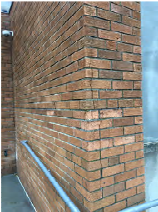
Restore Masonry at Lincoln High School
