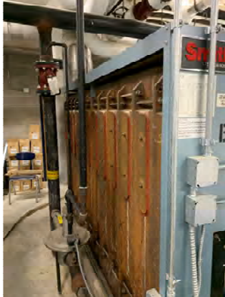
Boiler Replacement at Lincoln Middle School
